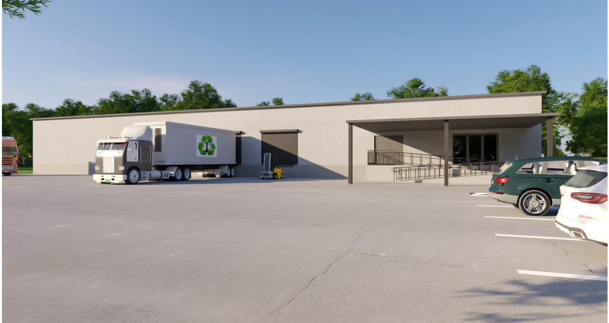
Front of building:
