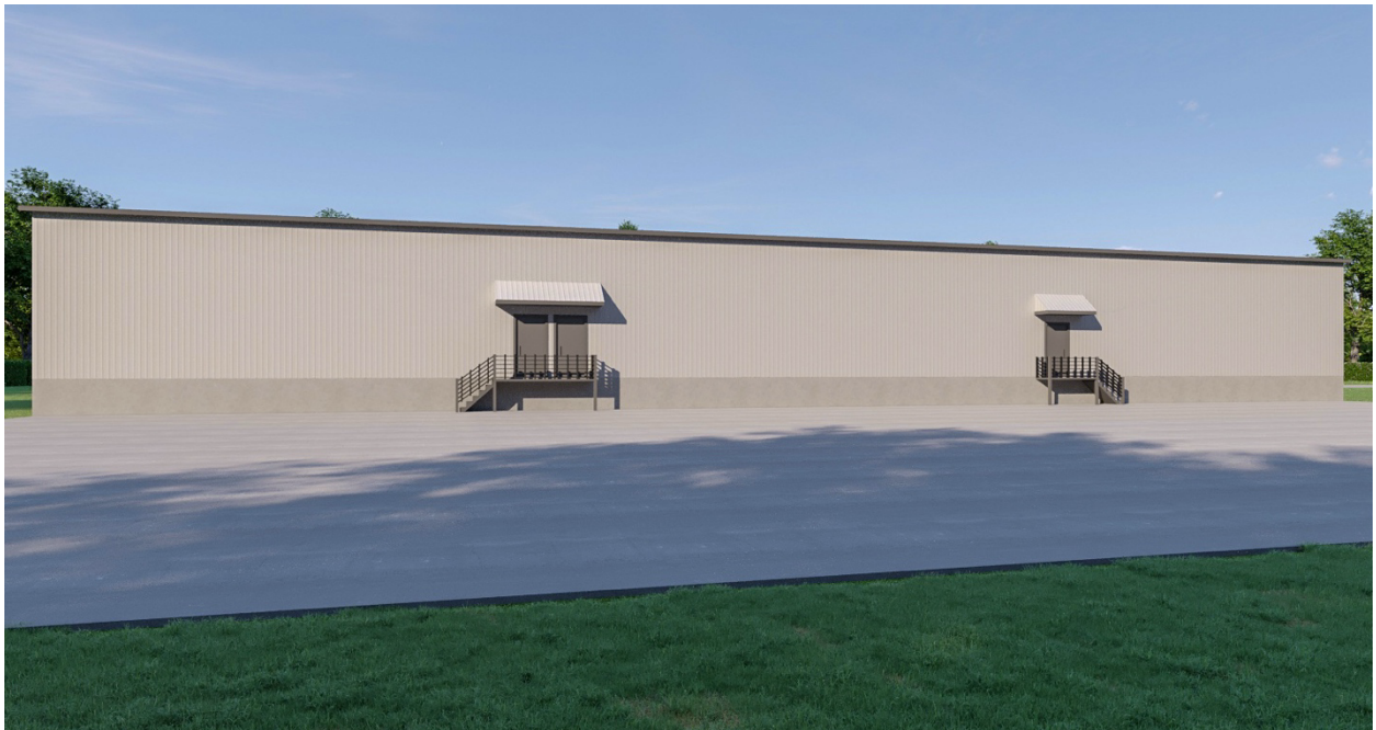
Back of building.
